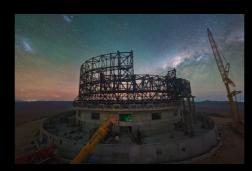
This image shows a webcam view of the construction site of ESO's Extremely Large Telescope at Cerro Armazones, in Chile's Atacama Desert. At the time the photograph was taken, in June 2023, engineers and construction workers were assembling the structure of the telescope dome.
